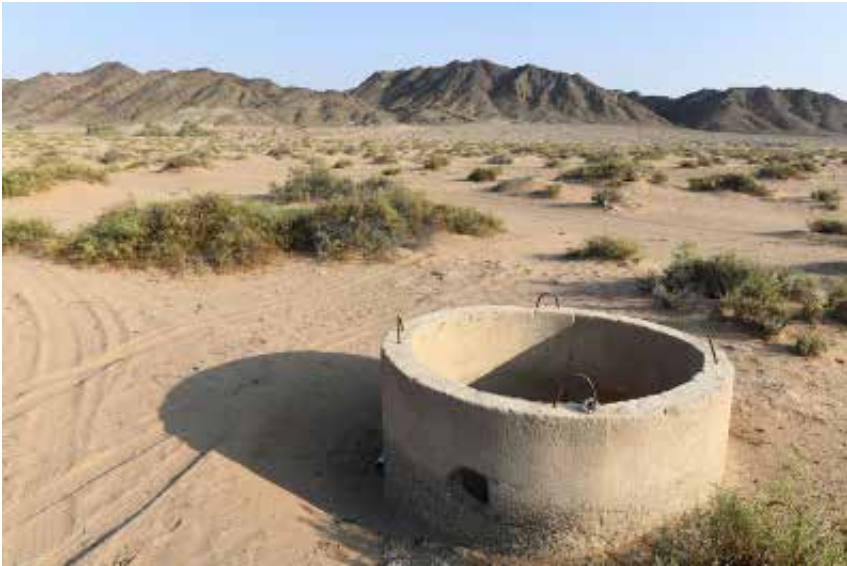
IMAGE 9. One of several water wells, recently enclosed in concrete, at Wadi al Aznam.
