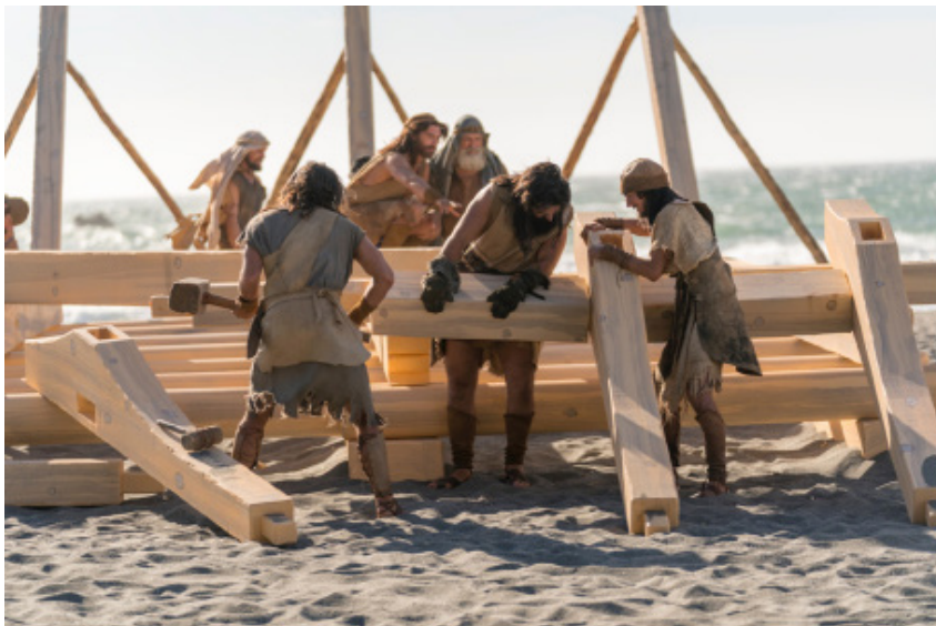
Figure 24. In the Church film of the Lehiite exodus, admirably accurate in most regards, Nephi's ship is built using the mortise and tenon method, with lashing suggested in various later glimpses while sailing. Image available at https://www.churchofjesuschrist.org/media/image/brother-ship-f608f8b .
